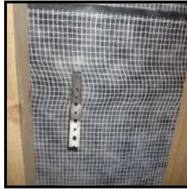
From attic cut a neat line in felt above holding batten to feed strap through
