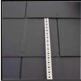
Slide stainless steel straps up between roofing material. See spacings pg 8.
