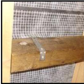
If batten is too light for fixings install a noggin between rafters and screw fix securely
