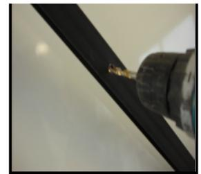
Drill 6.5mm holes in vertical struts in required locations (within parameters indicated in red on page 8)
